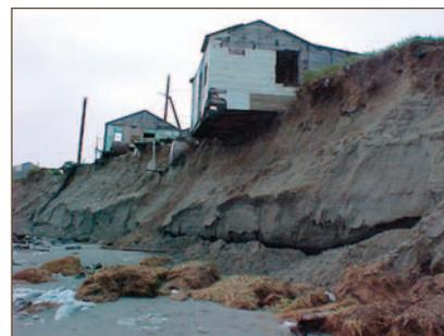
*Permafrost coasts are vulnerable to thaw subsidence and subsequent wave-induced erosion. Coastal erosion problems are an extraordinary challenge to arctic communities such as Barrow, Wainwright, Kivalina, and Shishmaref (above). Photo courtesy of Luci Eningoewuk and Native Village of Shishmaref.*
