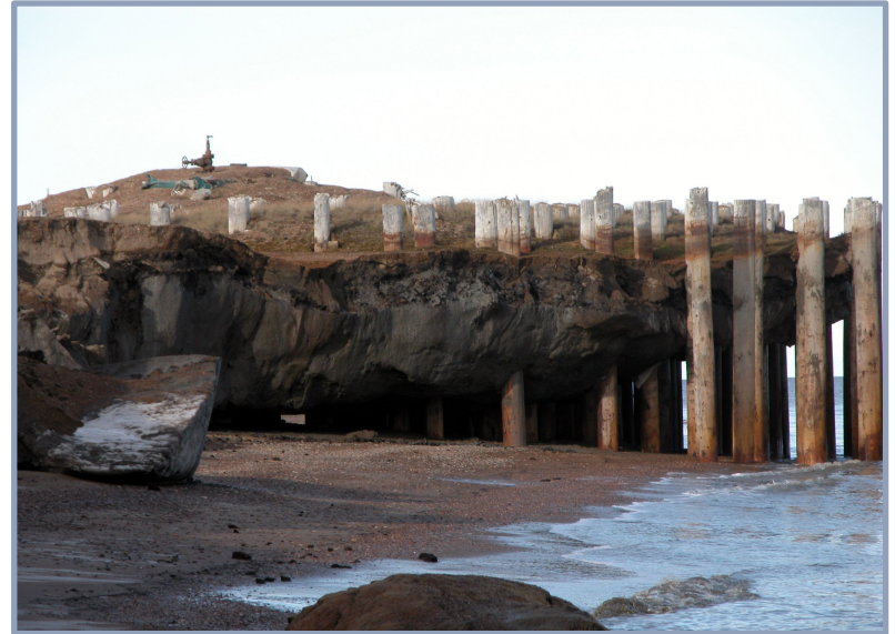
Oil and gas infrastructure Mitigation of several wells
