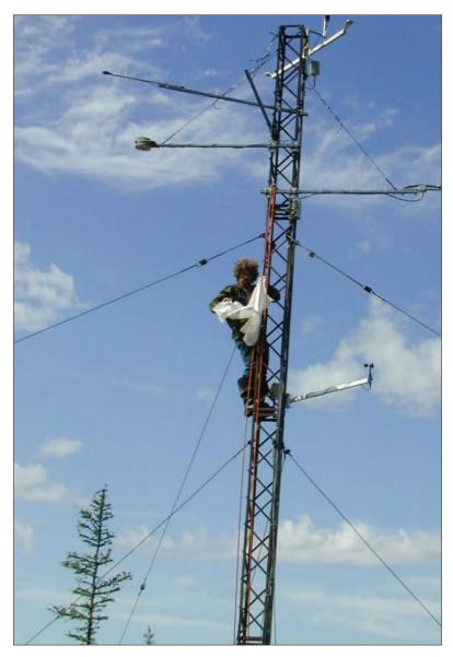
Sergei Zimov finishes installing instruments on an eddy flux tower near the Northeast Science Station in Cherskii, Siberia. Photo courtesy of VECO Polar Resources.
